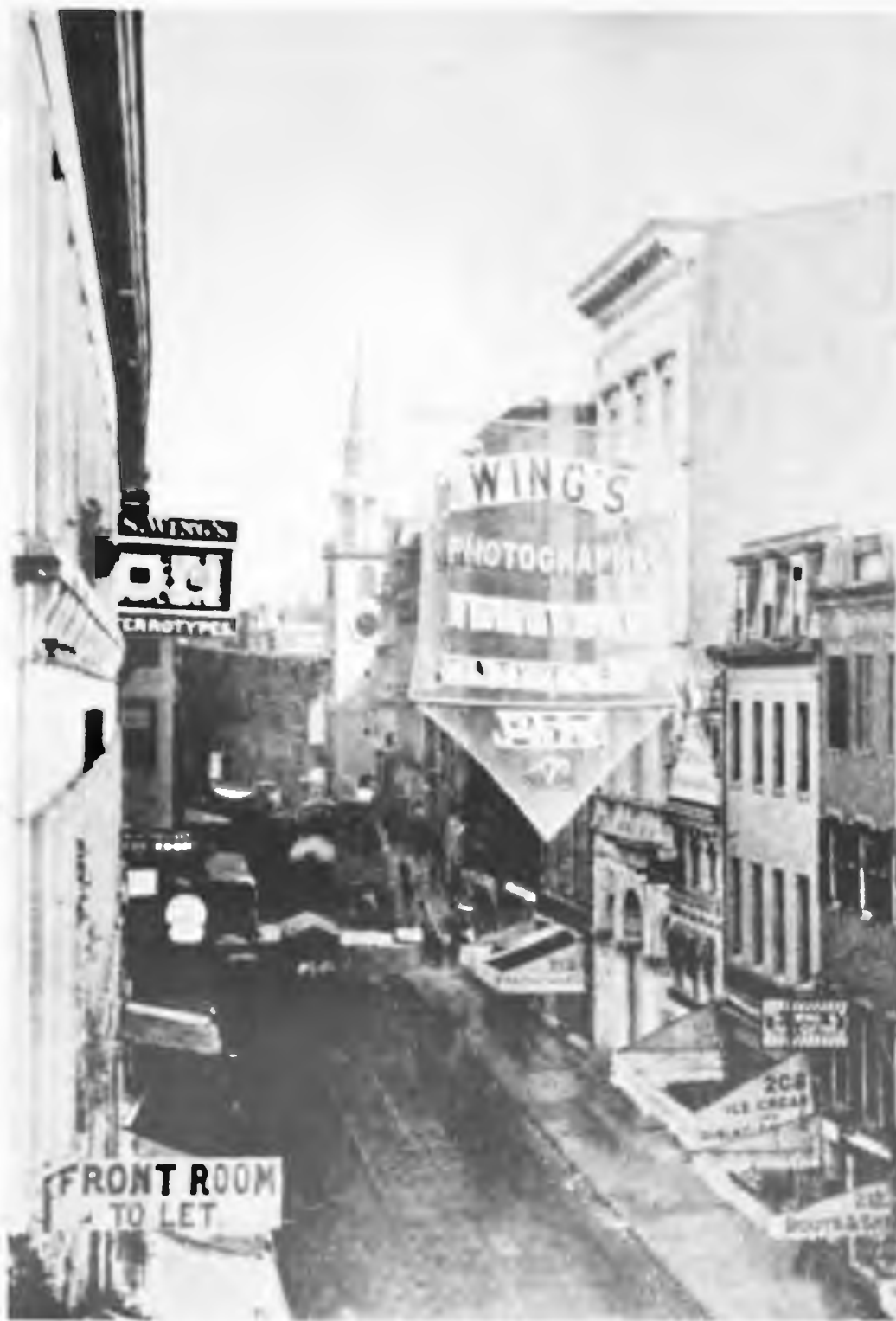
This view of Washington Street, taken around 1870 and enlarged from one side of a stereo card, shows two of Simon Wing's advertising signs for his studio at the 257 address. The large banner suspended over the center of the street was one of wing's non-photographic patents. Cut-out letters were attached to a cloth mesh enabling the banner to resist blowing in the wind.
